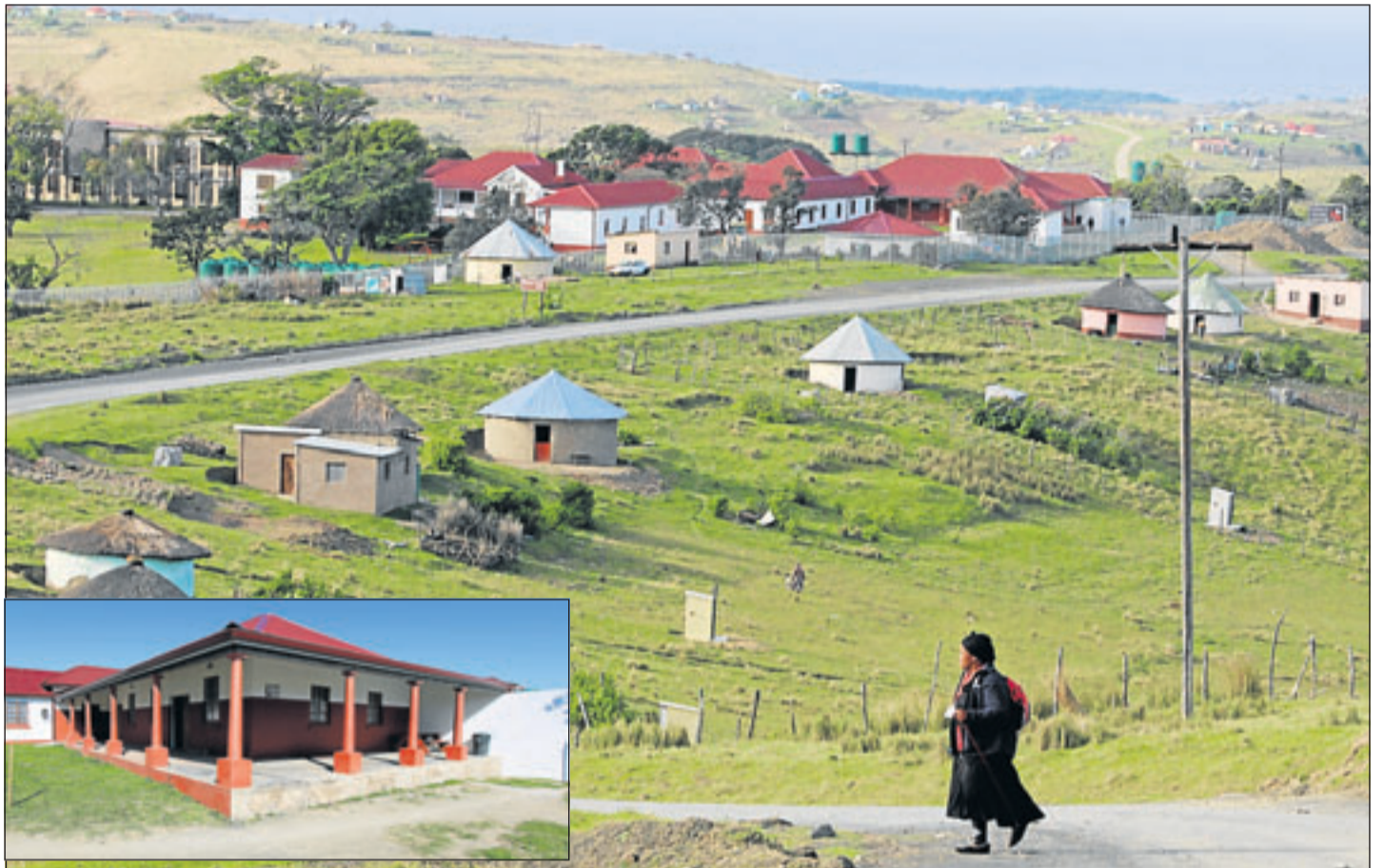
NEW HOPE: The Donald Woods Centre, which includes the old family trading store (inset), accommodation and training facilities, forms a vital part of the foundation set-up in the former Daily Dispatch editor's rural Hobeni home
